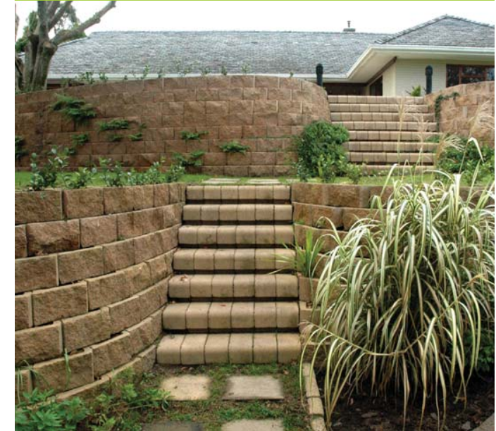
Two access stairs connect all the levels
